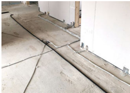
Rohinstallation Elektrik
